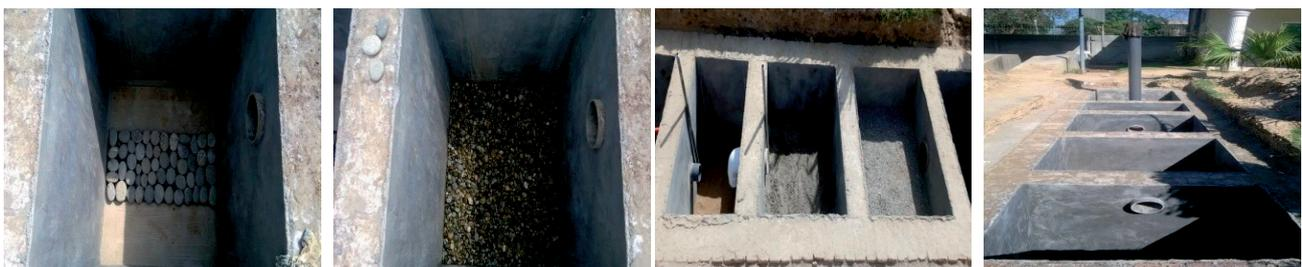
Fig. 3. Stepwise execution of Groundwater recharge well at PCRWR, Lahore.
