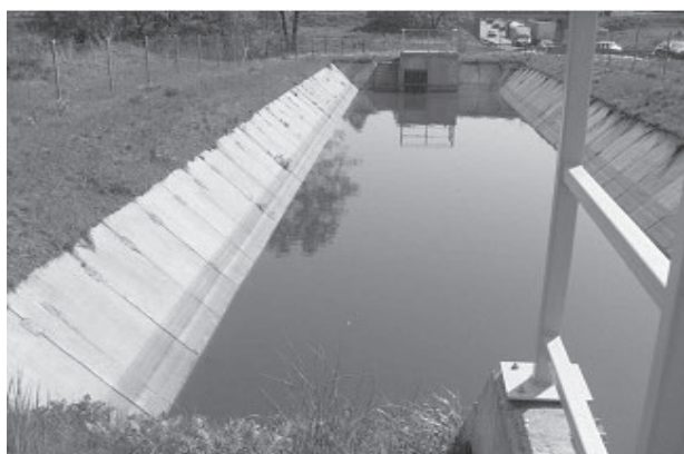
Fig. 2. Retention reservoir no 3 by the Kraków-Tarnów road (Photo A. Wałęga).
