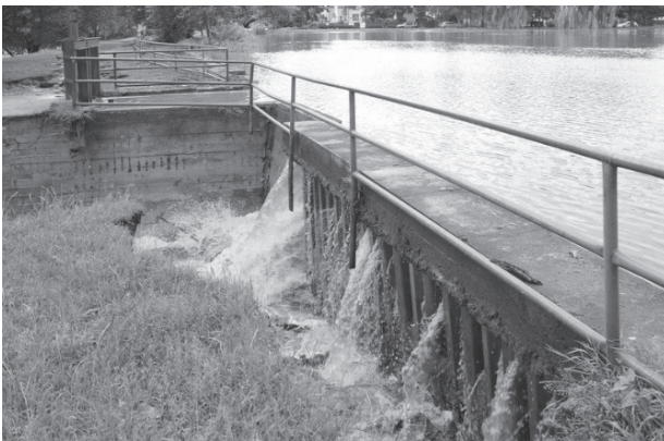
Fig. 3 Tank No.4 during floods on 14-15 July 2016 [11].
