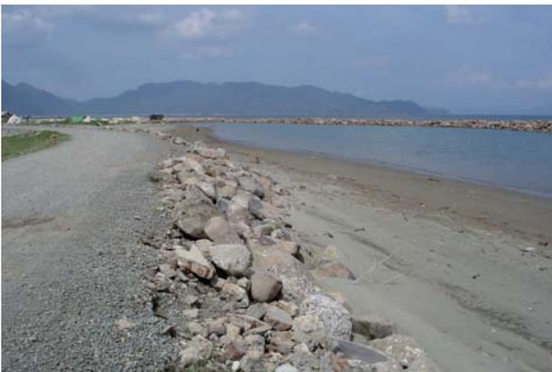
Fig. 2. Deah Geulumpang Beach in its early stage of recovery ceased to recover further when enclosed behind a rubble seawall that stretches from the east of the town to the Alue Naga Floodway Channel, March 2007.
