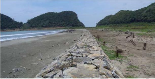
Fig. 16. South of Ujung Riteng, the beach is recovering and wide enough for protecting the road. A rubble seawall constructed up the headland in the south is unnecessary and interferes with beach recovery, March 2007.
