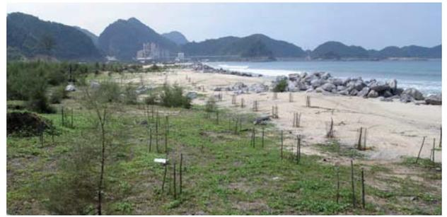
Fig. 17. North of the cement plant, Pasijalang Beach has recovered well enough to have casuarinas planted on its backshore and is used for local recreation. The construction of a rubble seawall almost along the berm crest would not be useful, March 2007.
