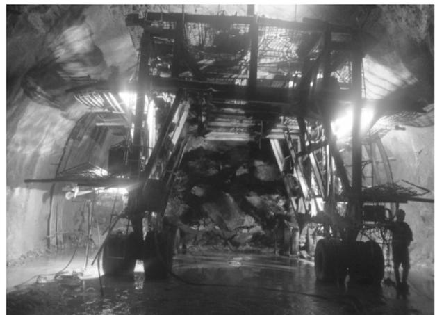
Fig. 1. Actual situation of a collapse in the tunnel.
