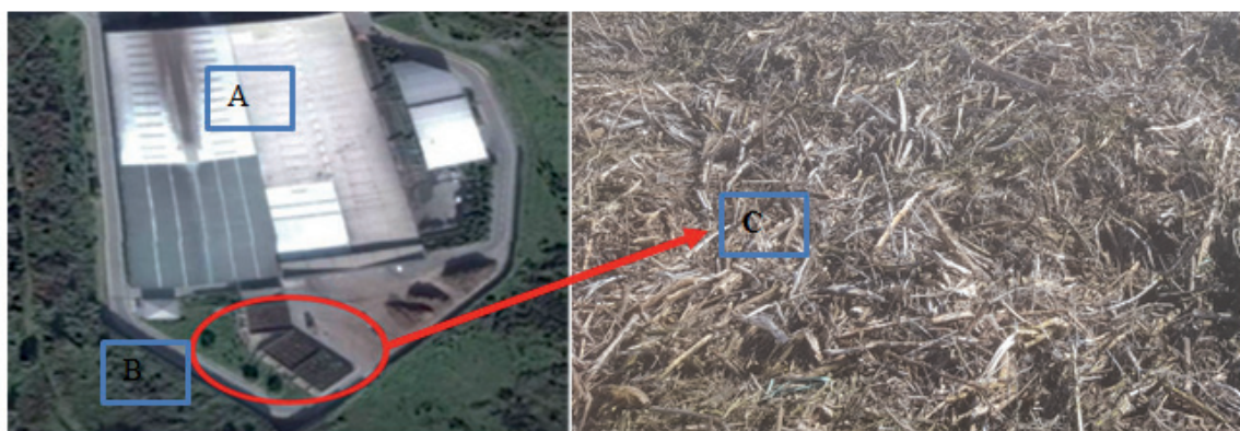
Fig. 1. A) Layout of composting and recovery plant (41°13'N and 28°49'E), B) Biofilter units, and C) Packing materials in the biofilter unit (woodchips).
