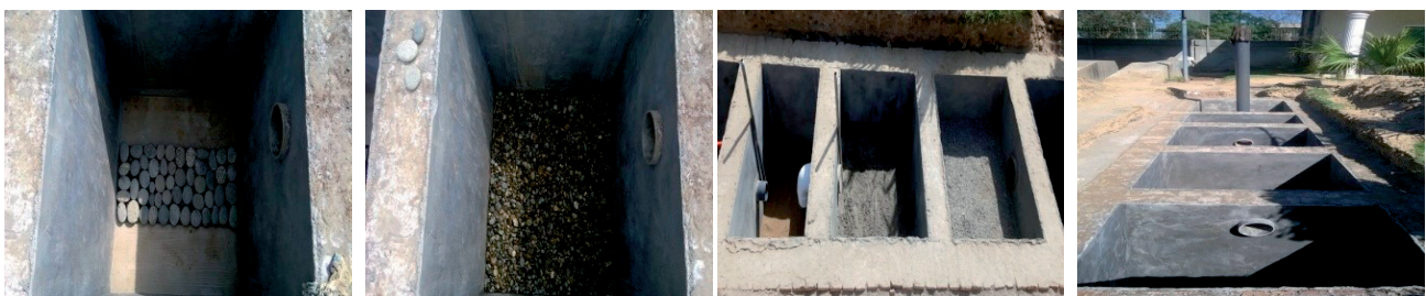
Fig. 3. Stepwise execution of Groundwater recharge well at PCRWR, Lahore.
