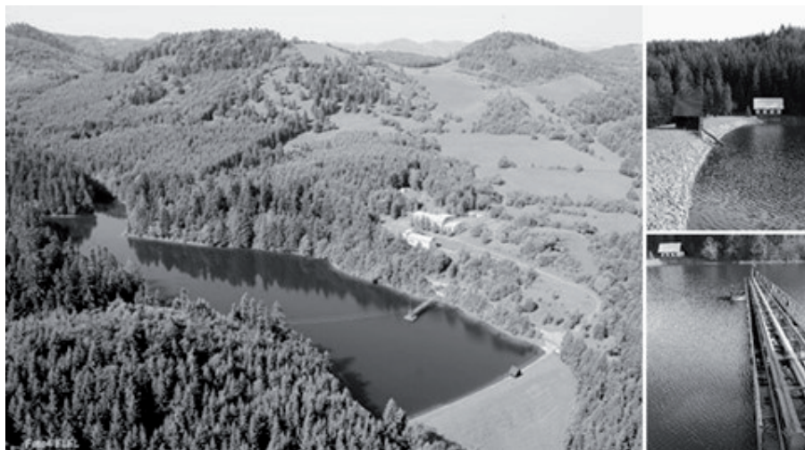
Fig. 2. A view of the Rozgrund water reservoir and the WTP Rozgrund (above the reservoir).
