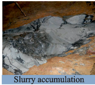
Fig. 2. Slurry accumulation.
