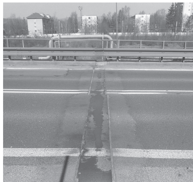
Fig. 1. Bridge joint – a source of specific sound.
