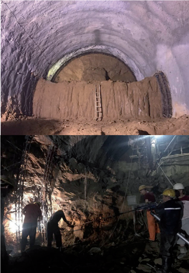
Fig. 2. Photographs showing the construction site.
