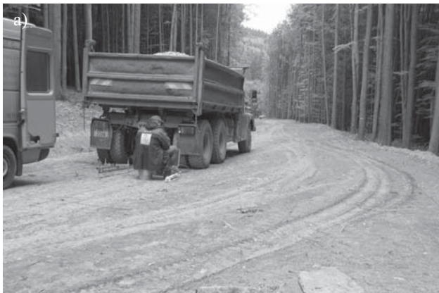
Fig. 1. a) Forest road “Kultury” – tests in construction
